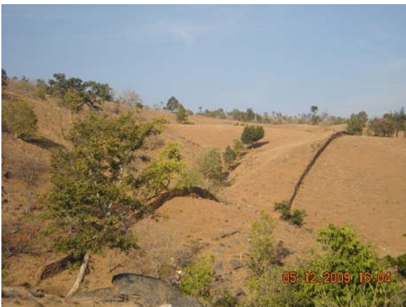
View of newly erected boundary wall in Lildi JFM
